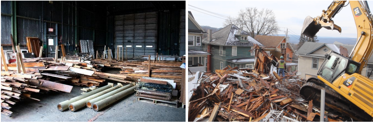
Figure 4: Photos by Joseph McGranahan (left), Melody Chen (right), Circular Construction Lab A visual to contrast the process (top) and aftermath (bottom) of deconstruction (left) and demolition (right)
