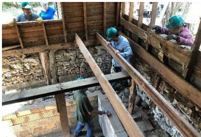
Photo by San Antonio Reuse
