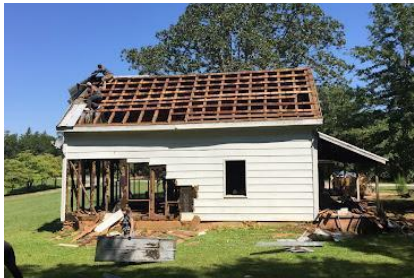
Photo by Demolition Deconstruction
